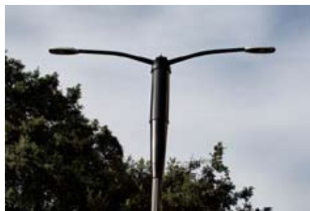
Smart light poles in San Jose combine small cells and sensors.
