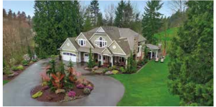
WINE COUNTRY ARCHITECTURAL MASTERPIECE Authentic beauty in an exquisite setting—Hollywood Hill’s premier estate built by “Street of Dreams” esteemed builder, Parmenter Homes. $2,368,000. windermere.com/mls/902377
